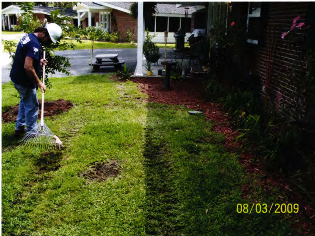
Picture 2: Site after completion of work.
